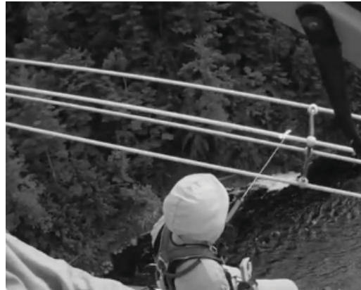
(b) Inspection of high voltage power cables ( http://www.haverfield.com ).
